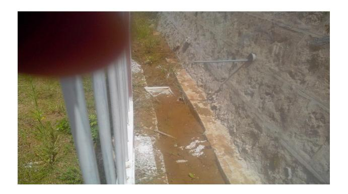
**8.** Side drain was blocked due to improper care and sluggish gradient.
