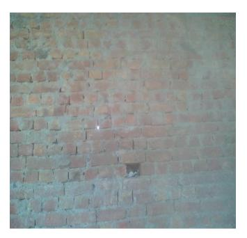
5. Quality of brick masonry work was very poor.
