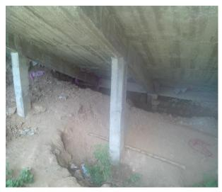
7. Strength and alignment of beams and columns seems poor.
