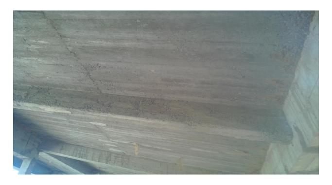
6. Honeycombing was observed in beams, columns and slab which shows the poor quality of workmanship.
